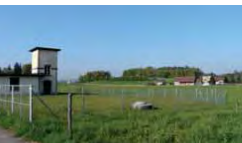
Pumpwerk in Lindau
