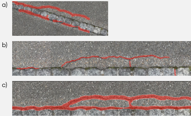
Figure 7: Predicted defect viewed through OCL. Comparing zoomed views focussing on the same location of the runway. Sub-figure a) shows M3 results which are aligned so that north is at the top; hence, the image is rotated. M1 and M2 are aligned so that the main axis of the runway corresponds to the image orientation. Subfigure b) shows results for M1 (fine setup) and subfigure c) for M2 (fast setup). The real crack, which extends into the surface of the runway, is reliably detected in all three setups.
